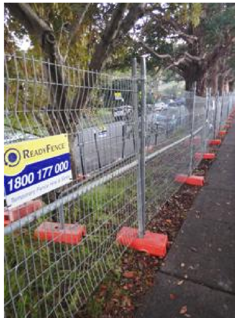
Example image of acceptable tree protection fencing measures to be applied. (1.8m high rigid metal fencing with appropriate lateral bracing)
